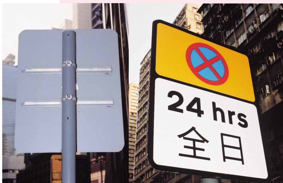
正在試用中的套入背槽式交通標誌。 New traffic signs with mounting channels at the back are being put on trial.
