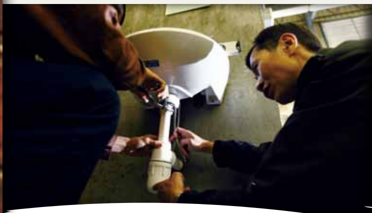
工艺人员指导青少年所员修理水喉器皿。 A technical instructor teaches a young inmate way to repair water pipe utensils.
